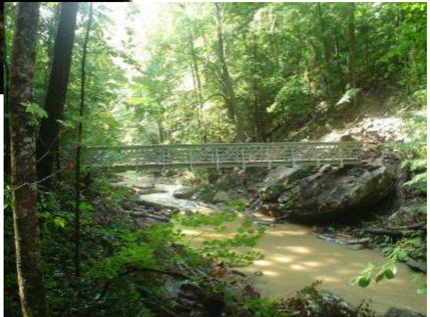
Little Possum Creek Bridge
