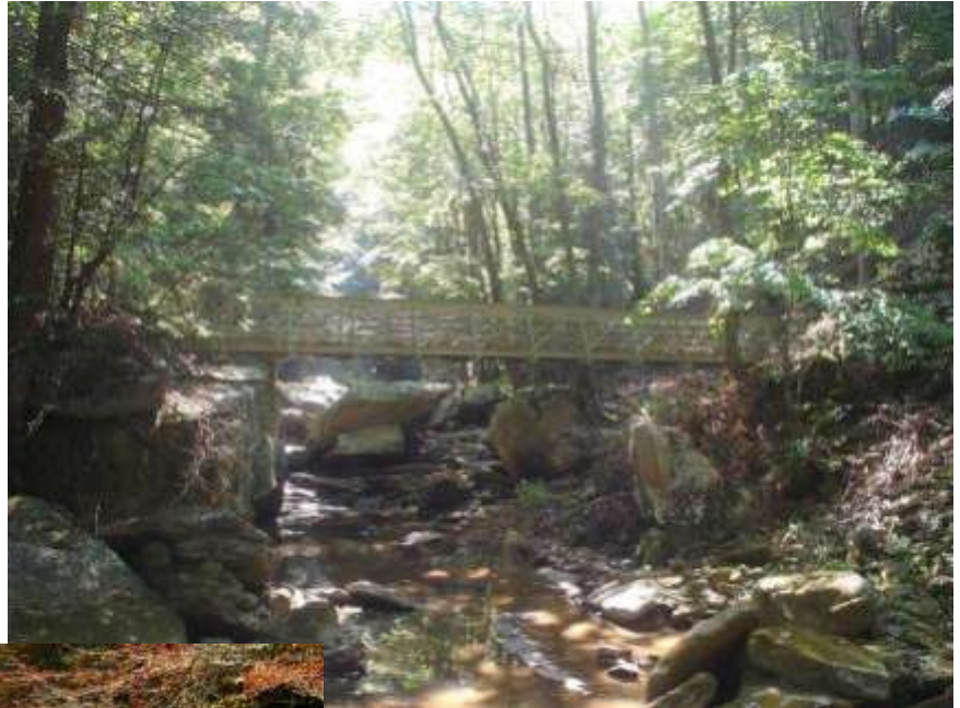
Big Possum Creek Bridge
